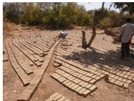
Just some of the 100 000 plus bricks made by the community
