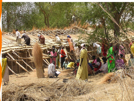
Women working on the new roof at the school in late 2009
