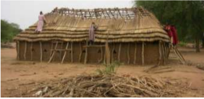
Women rethatching the roof on the 2007 built classroom at Wäramoth Primary
