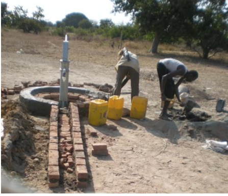
Community members finalising the laying of concrete around the bore hole in Mabok.
